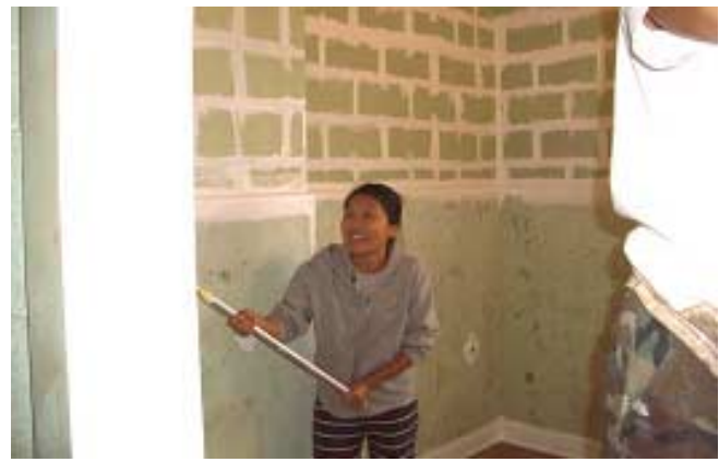
Left & Right – We're getting into it! – Stanza 2: Cleaning and preparing the interior walls for paint. These volunteers did this before! Notice how they've painted the mortar joints prior to applying paint by roller.
