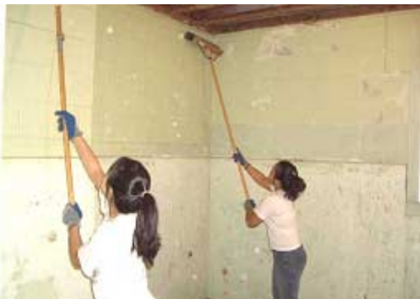
Left & Right – We're getting into it! – Stanza 2: Cleaning and preparing the interior walls for paint. These volunteers did this before! Notice how they've painted the mortar joints prior to applying paint by roller.
